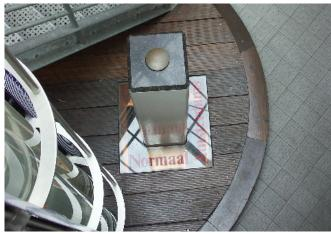
as far as the second sand layer. On top of the pillar is the bronze N.A.P. reference point. The top is precisely at the Normal Amsterdam Level, i.e. the zero level. The reference point was set at correct height on 18 May 1988 by the Minister of Transport, Public Works and Water Management.
